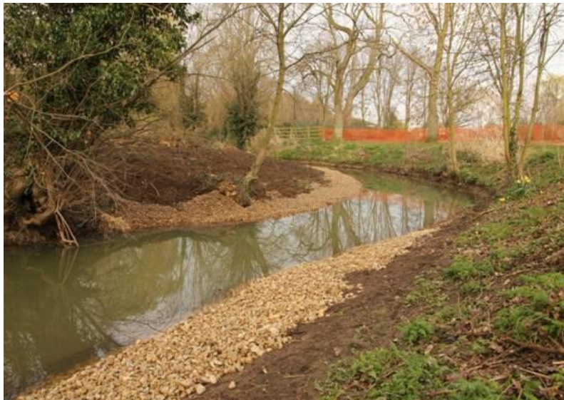
Gravelled berms immediately after construction
