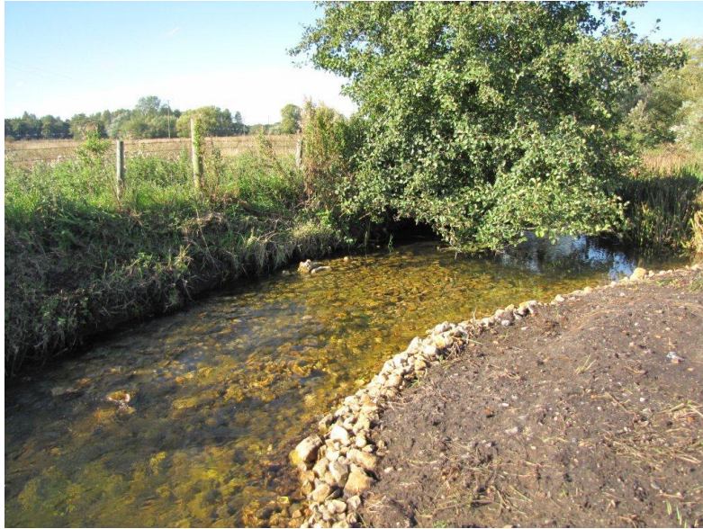
Gravelled berms immediately after construction
